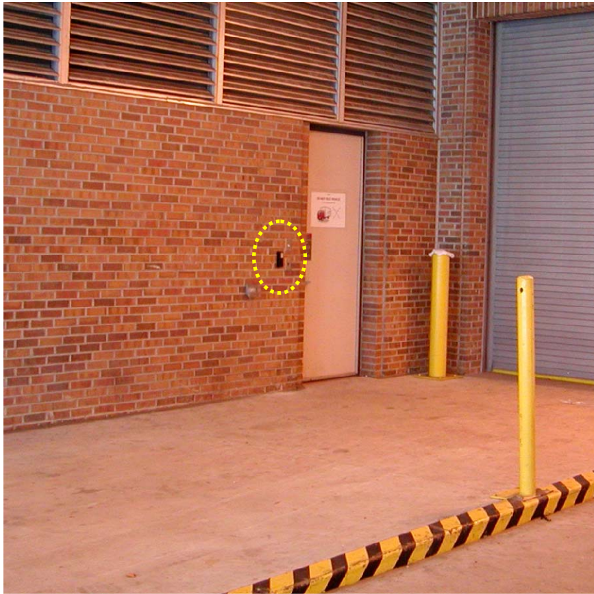
BuckID Card Reader Installation at West Loading Dock Entrance
